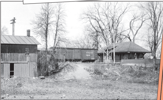
ABOVE: The "Peanut" crossed the Erie Railroad at Golah, the NYC station can be seen at right.
