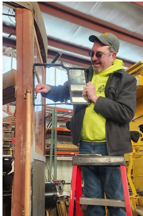
RIGHT: New volunteer Karsen Nunn helped re-install the handbrake inside the cab of Rochester Subway Car 60 on January 11. The chain has been reconnected, and the brake functions again as intended. KARSEN NUNN PHOTO
