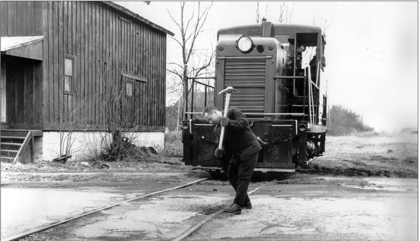
ABOVE: Conductor John Iler uses a pickaxe to clear the flangeways at Stone Hill Road in Lakeville so the very first LA&L train could proceed on April 7, 1965. GE 44-tonner No. 10 was acquired second-hand from Vermont Railway, and was sold to a Cargill elevator in Ohio in 1978. GENE BLABEY PHOTO
